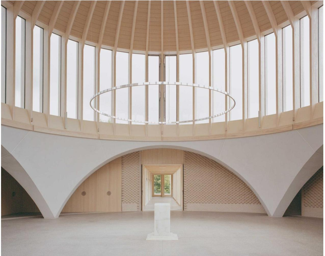
The acoustics within this space were also tricky, due to its composition from four different materials set at various angles. As such, the use of materials and treatments internally also became very technical: the use of textured brick to scatter sound and perforated ash (the pinholes so tiny they're only visible up-close) acting in place of acoustic baffling. The sound is surprisingly even from every part of the room.
