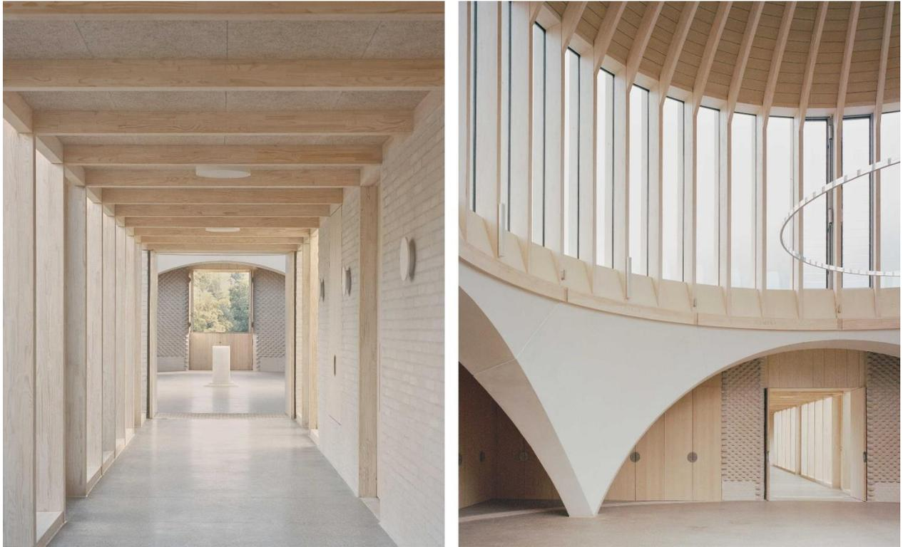
A 12m-diameter circle determines the inner temple, helping focus the congregation's attention onto a central altar. The space is enclosed by a pendentive structure supporting a lantern and dome, akin to those seen in Byzantine, Renaissance and Baroque churches, with arched openings to the cardinal points in the pendentive. Supporting a circular timber and glass lantern above, this structural element's form is modelled as a three-dimensional expression of the energy lines crossing the site.
